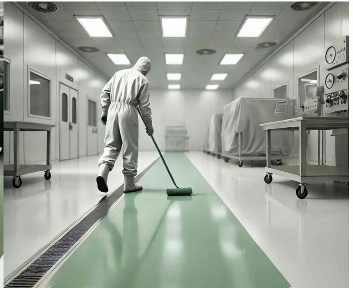
FLOORS & WALLS INCLUDING CONCRETE, TILES, STONE
